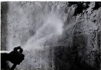
Wet wall down with spray from garden hose.
